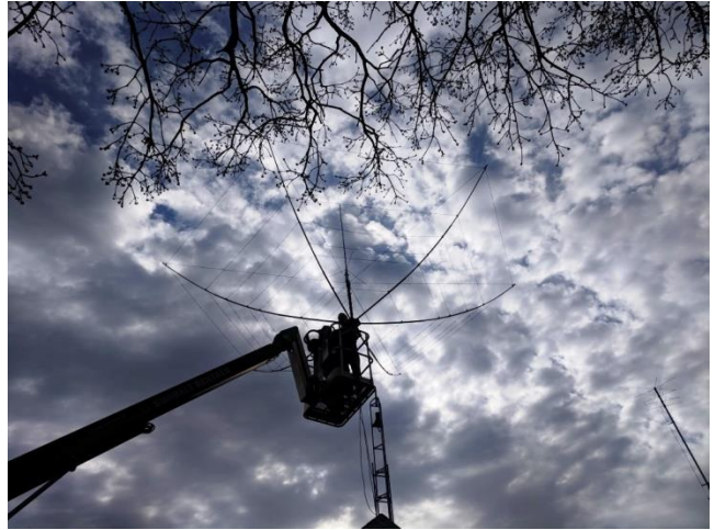
Daniel placing the HEX BEAM on the tower
