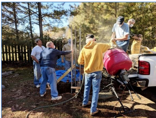
"Yep. Its vertical." says K4MWC. K4LDC & K4ZMW agree. K4ZEC, KM4VTE & K4BBH mix more concrete.
