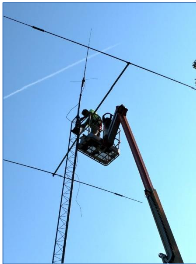
John – K4SSE disassembling the tower and antenna
