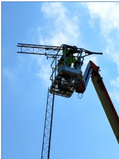
John – K4SSE disassembling the tower and antenna
